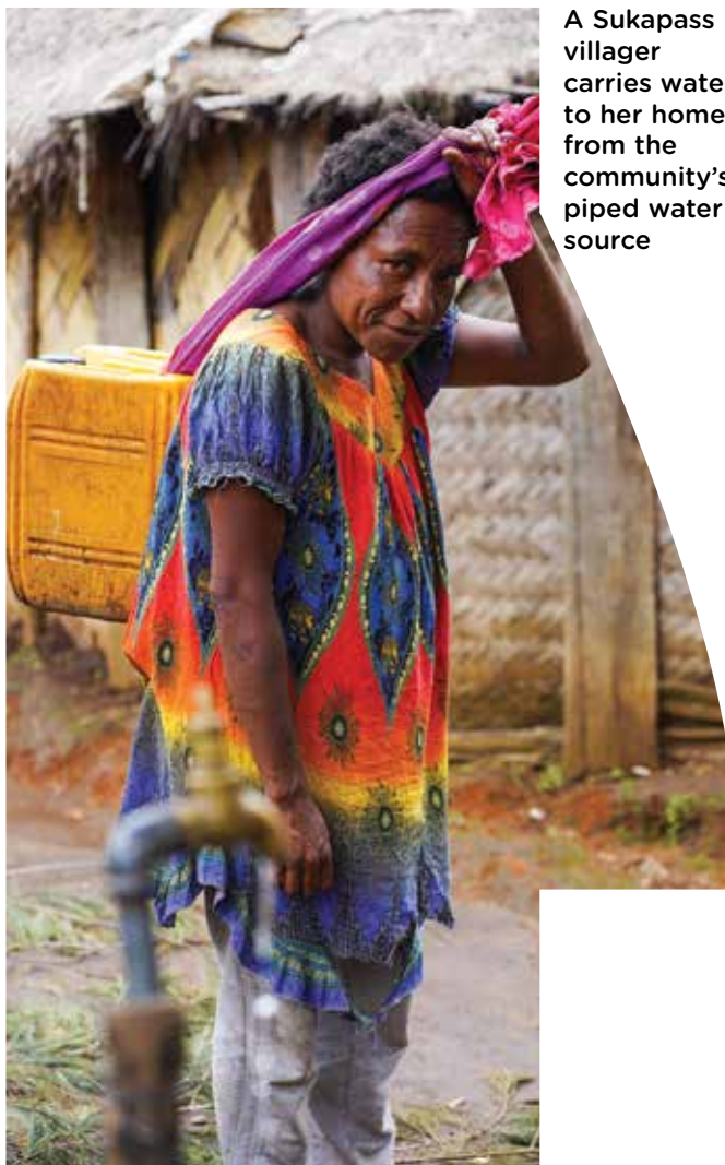
Ihato Bery from Sukapass village is delighted to have fresh drinking water from the water pipe newly installed in her yard
